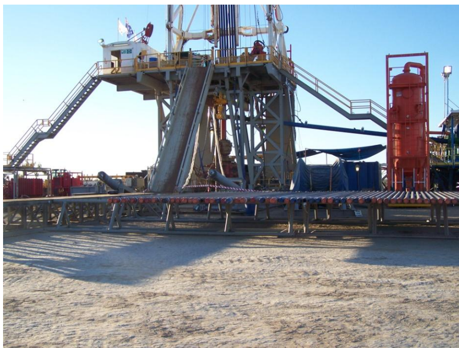
7" casing racked beside Rig 100 at Jolokia 1
